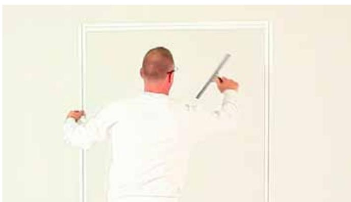
Complete a second cleaning using mild soap and water to ensure the window is completely clean.
