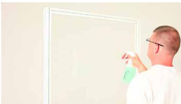
Surfaces to which the material will be applied must be thoroughly cleaned from dust, grease or any contamination that could affect the adhesion of the material.
