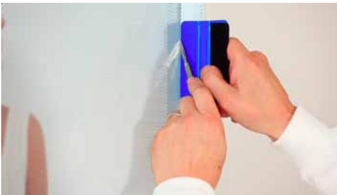
Cut the graphics back from the edge of the window by 1-3mm to ensure reliable edge adhesion.
