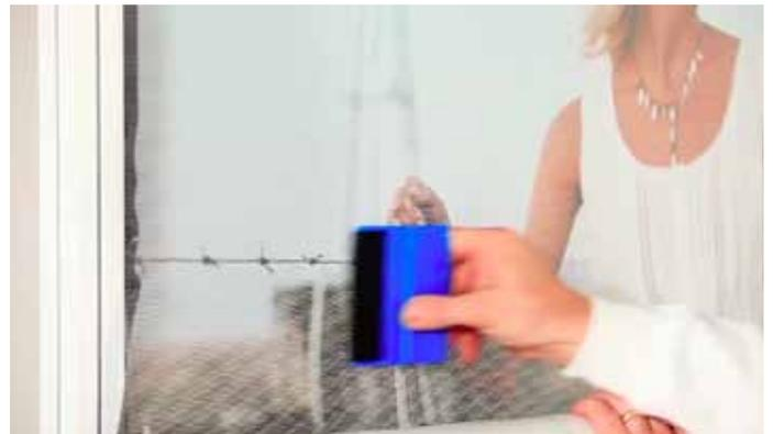
Otherwise, just squeegee down evenly, handling the graphic with care, and ensuring that no bubbles are trapped beneath the graphics.
