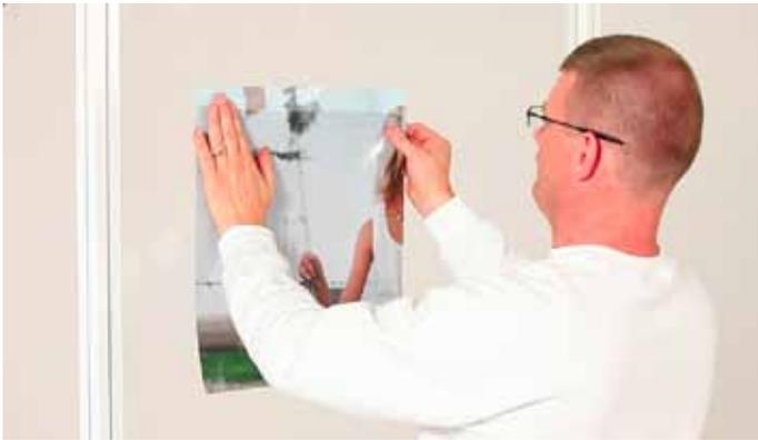
Use a butt joint, not an overlap joint. Apply the first panel.
