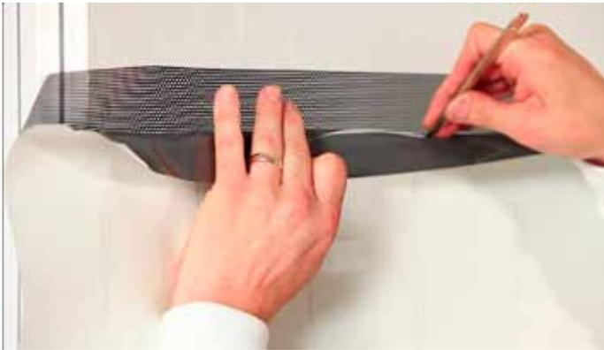
Apply dry using a plastic applicator with a low friction sleeve. Avoid touching the adhesive, especially at the edges and corners. Cut away the top 25-50mm of the liner.
